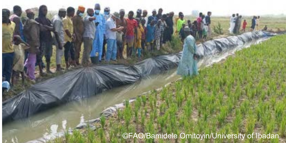
Figure 2: Plastic lining as an initial adaptation measure to prevent water seepage.
